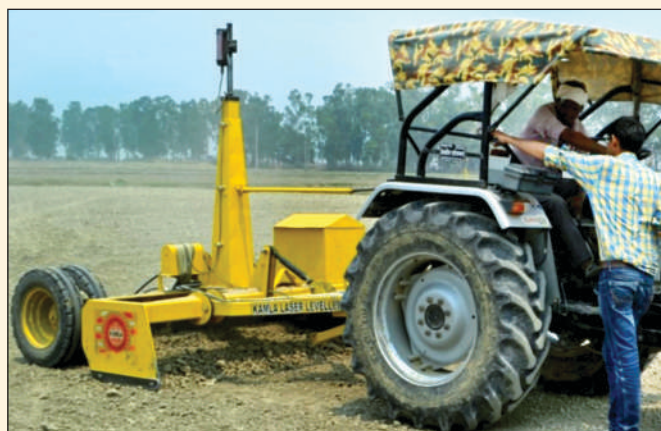
Land levelling through laser land leveller in field
